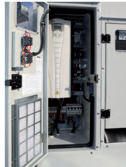
Pressure regulation through inverter brand ABB IP 55, protected by safety sensor on door openable.
